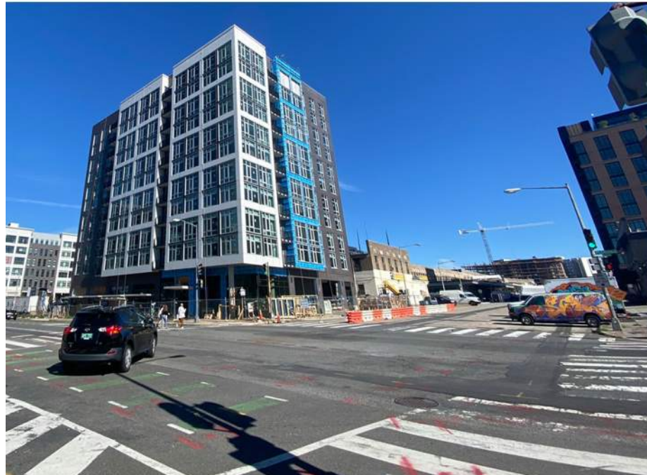
4. 5th St NE & Florida Ave NE_ 12 Floors
