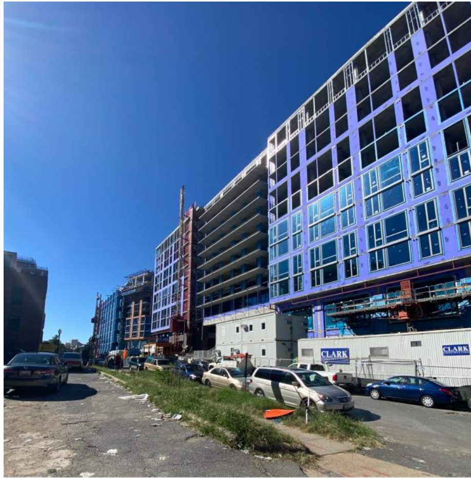
7. 1200 Third St NE_ 12 Floors Plus Penthouse
