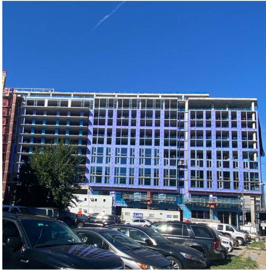
1. 1200 Third St NE_ 12 Floors Plus Penthouse
